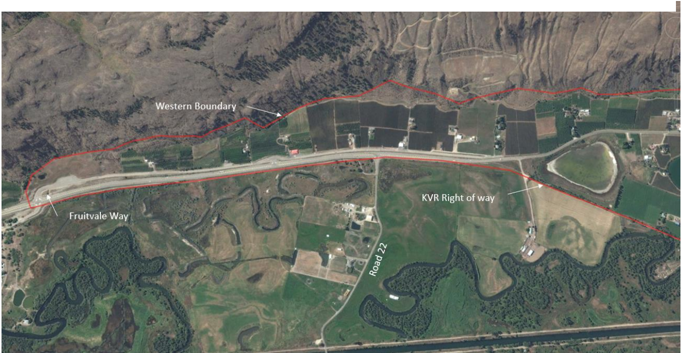
Figure 5. In the southern extent, the GI becomes quite narrow as the floodplain of the Okanagan River extends right to the edge of the highway.
