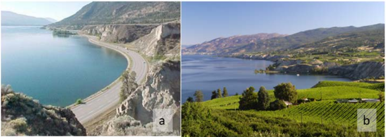
Figure 8. Exposures of well-preserved deposits of glaciolacustrine sediments can be seen along Hwy 97 south of the Summerland Research and Development Centre (a). These deposits are composed primarily of silt and fine sands. Much of the Summerland Lakefront GI can be seen in the photo looking south toward Penticton (b). Agricultural land in the foreground sits on a glaciolacustrine terrace.
