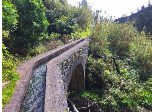
'Levadas' are the main irrigation methods- 2150 km in length, 40 km in tunnels
